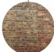
Existing engine house brickwork
