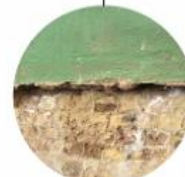
Existing coloured render and brick
